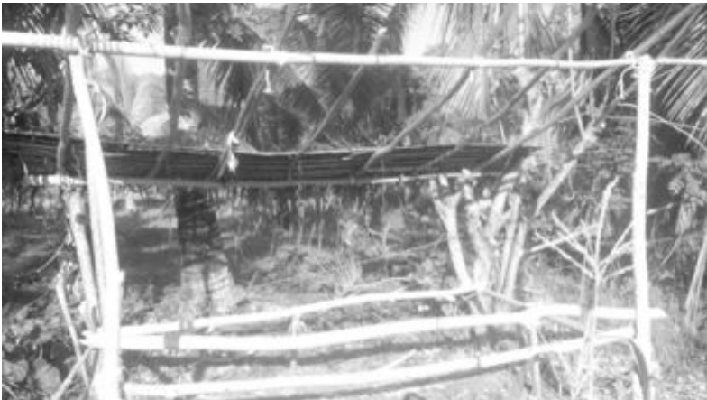
Figure 9. Nanay Soping's future home which is still under construction.
