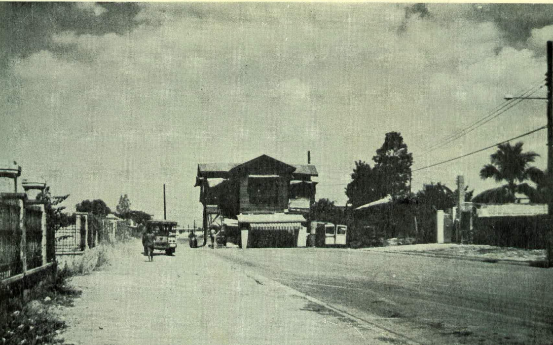
PLATE 2. House blocks road construction off Quezon Boulevard Extension, Quezon City. Resident's tenacious claim to ownership dramatizes conflict between individual and community needs.
